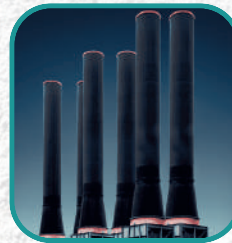
Boiler Condition Assessment
