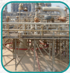
On & Off Stream Inspection Programs
